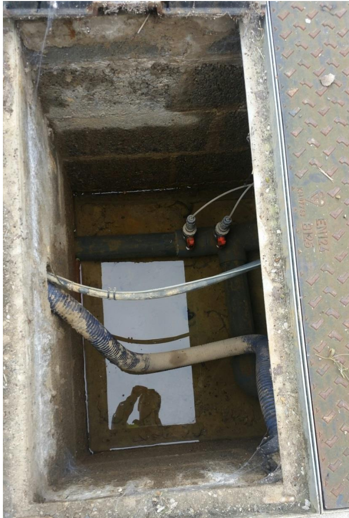
Photo 2. Redundant Sodium Hypochlorite Dosing Points on the Outlet of the Reservoir (note the chamber is partially filled with water)
