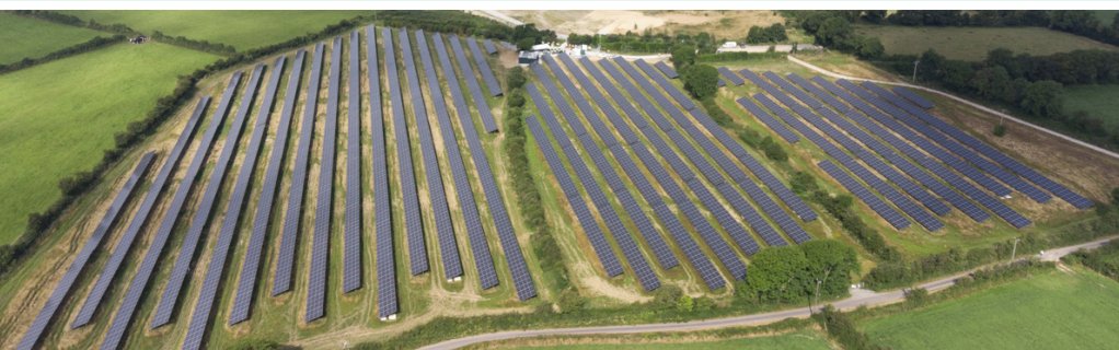
Solar Farm Installation at Licensed Site
