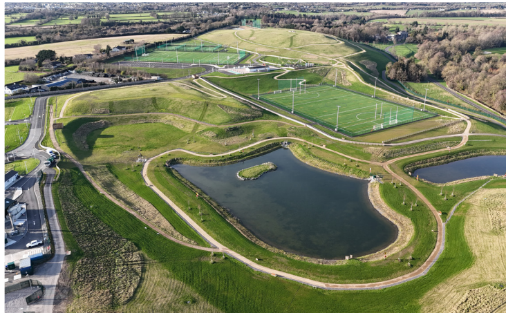
Remediated Kerdiffstown Landfill
