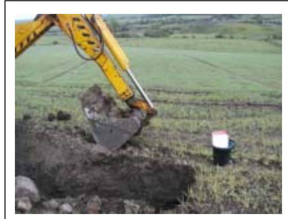
Plate 9: Mechanical Digger & trial hole (Photo: D. Kelly)
